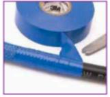
Starting at the line, take a few tight turns of tape down the application so that it covers the sleeving and extends about 1 1/2" on the application. Make sure the tape is smooth and tight. Cut the end and press down for a smooth finish. 3M 2242 Self Bonding Tape
